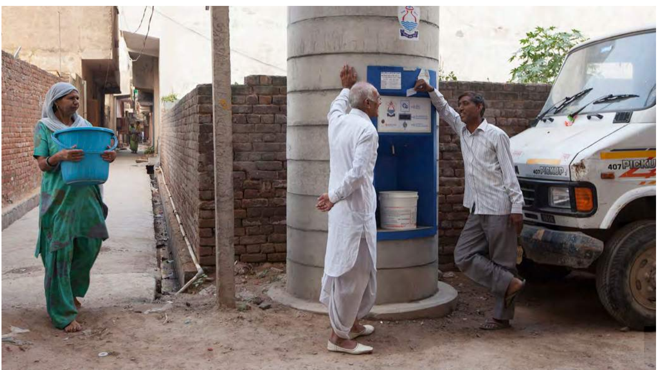
The solar powered vending machines installed by a for-profit social enterprise called Piramal dispense clean drinking water via a pre-paid smartcard to residents who have no access to water on tap in their homes. New Delhi, India. (Photo by In Pictures Ltd./Corbis via Getty Images)
