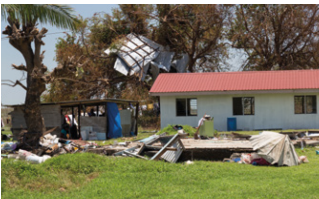
The effects of Tropical Cyclone Winston, December 2016.
